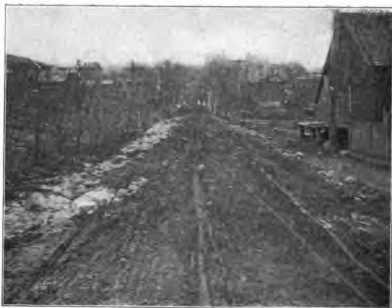
Stanhope and Newton road, Sussex Co., before improvement.
